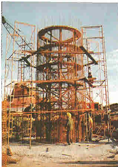
Rebar template cylinder reinforcing assembly.
