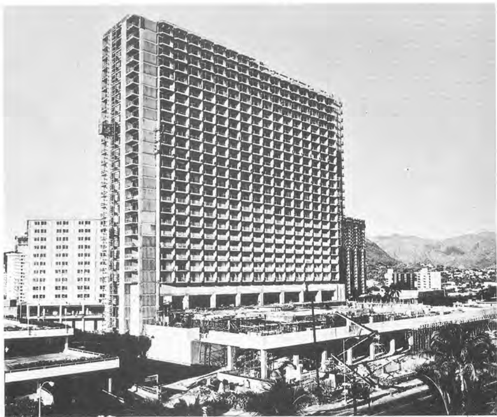
Fig. 1. Ala Moana Hotel in Honolulu, Hawaii, nearing completion.
