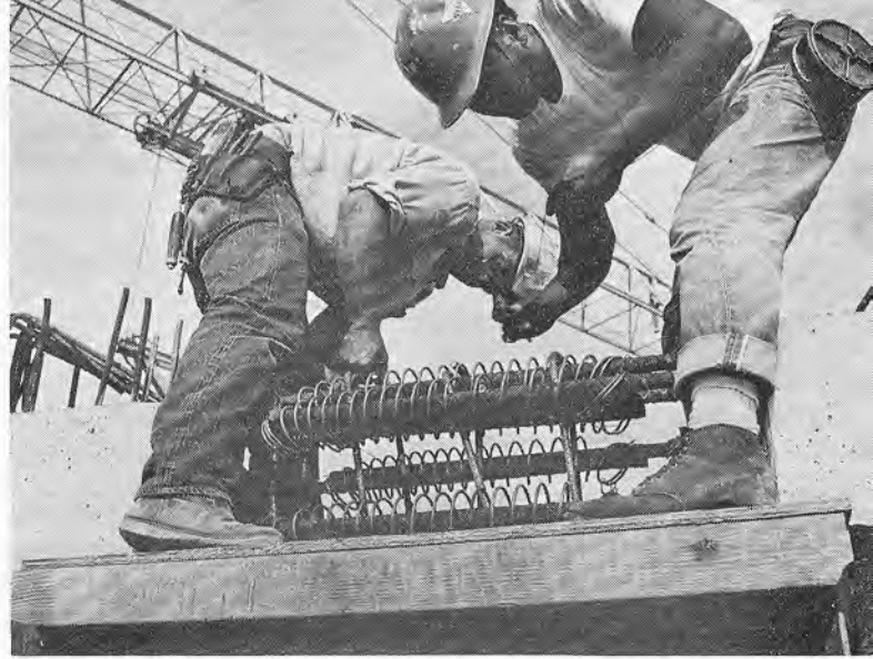
Steel coil is wrapped around rebar to increase bond of lapped splice used to join tree branches.
