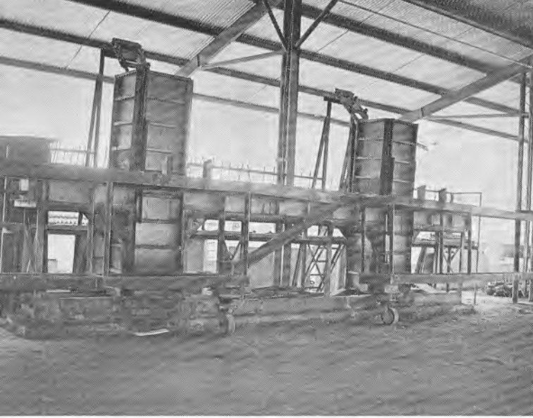
H-frames were cast in special forms in an upright position.
