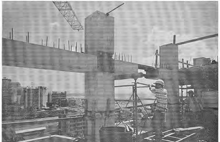
Tree being erected was supported on tubular shores with adjustable jacks.
