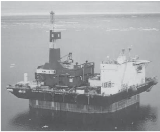
Fig. 3. Concrete Island Drilling System (CIDS) platform constructed with precast and prestressed concrete elements designed to withstand the severe ice-floe pressures of the Arctic. The CIDS platform replaces the building of gravel islands, which cost approximately $100 million to construct, whether oil was found or not. In contrast, the Concrete Island Drilling System cost only $75 million to construct and has been reused for the past 20 years to explore numerous locations along the north Alaskan coastline in the Beaufort Sea without showing any deterioration in the hull. In addition, it leaves no footprint on the seabed. The CIDS is presently operating along the east coast of Russia.
